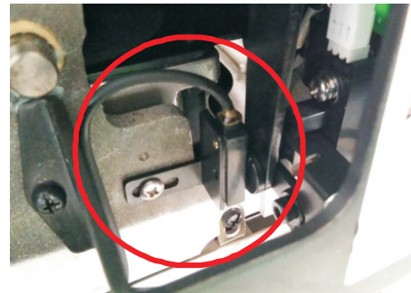
Fig. (14) After the Sensor Installation
